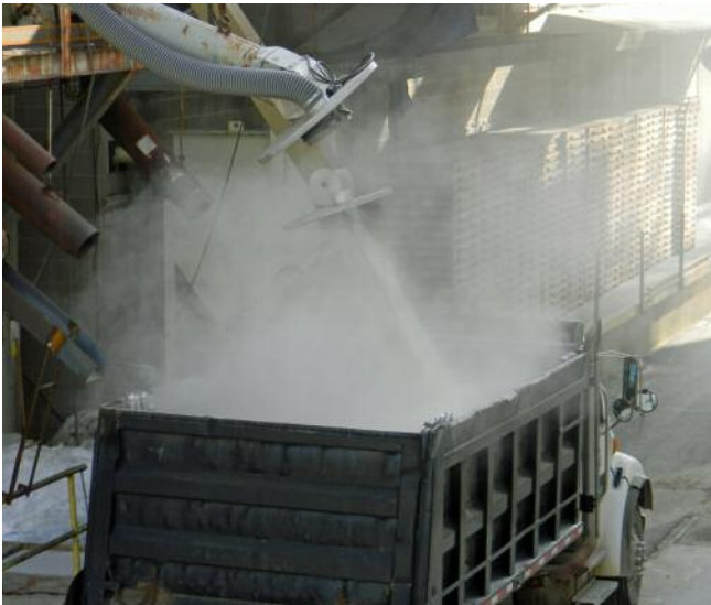
Before and after installation of the DSH System.
