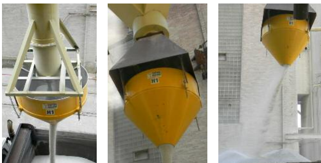
DSH installation and operation.
